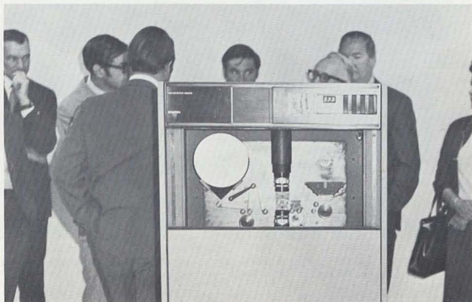
THE PROTECTIVE cover of the printer slides away to reveal some of the machinery. The white disc is a reel of microfilm.
